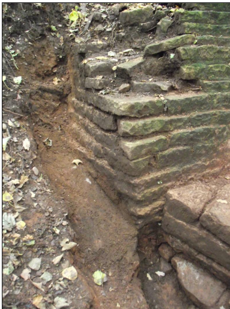
Plate 2: Eastern wall of sluice, partially destroyed. Pinkish clay has been used to fill this gap. Looking north east (L. Binns 2015)
