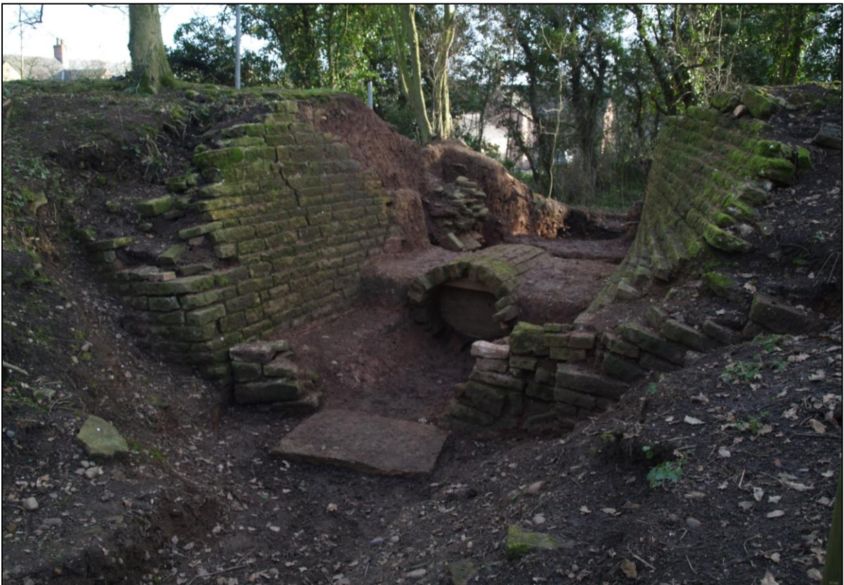
Plate 11: The brick culvert running parallel to and the same length as the sluice walls. Looking south east (S Walker 2015)
