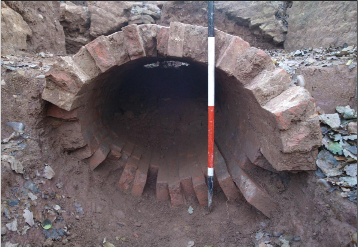
Plate 10: Profile of the culvert. Looking south (S. Walker 2012)
