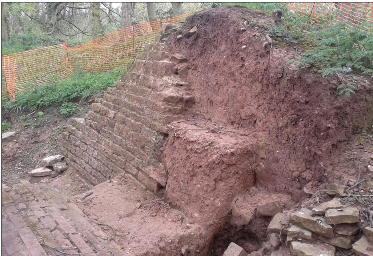
Plate 2: Eastern wall of sluice, partially destroyed. Pinkish clay has been used to fill this gap. Looking north east (L. Binns 2015)
