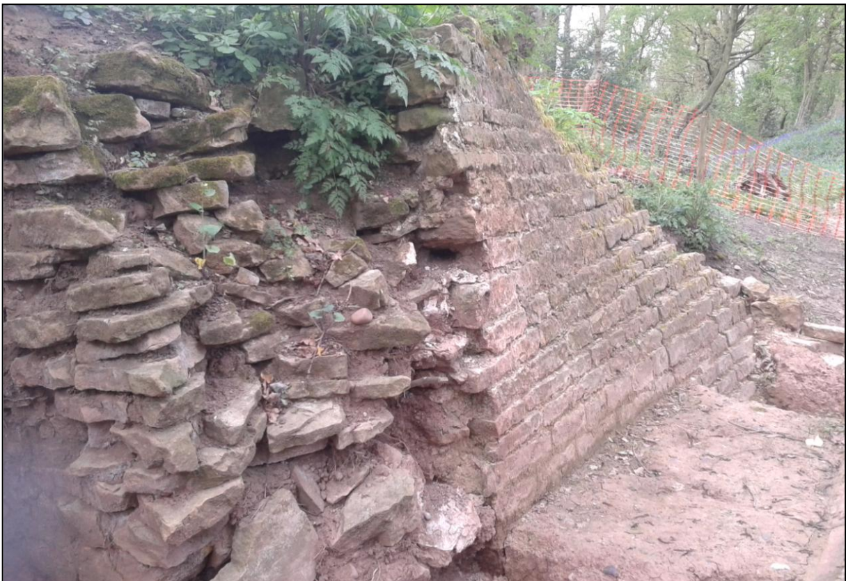
Plate 5: Western wall of sluice, the southern end, where the sluice face seems to be keyed in with the cross wall. Looking north west (L. Binns 2015)
