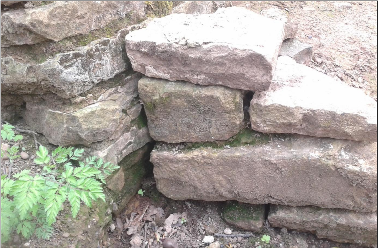
Plate 6: Dry stone northern wall [0009] abutting the eastern wall of sluice. Looking south east (L. Binns 2015)
