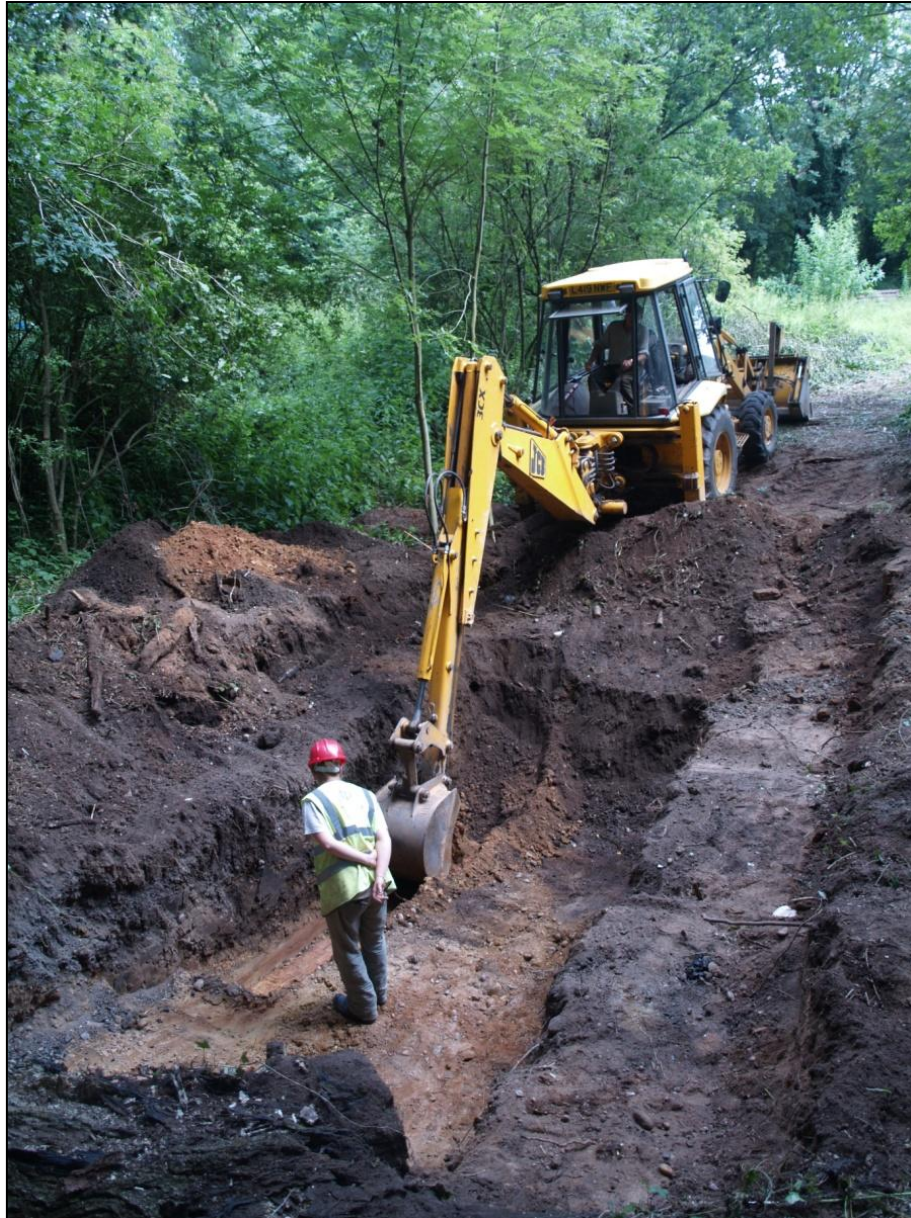
Plate 1: The excavation of the trench. Looking north east (S. Walker, 2014)
