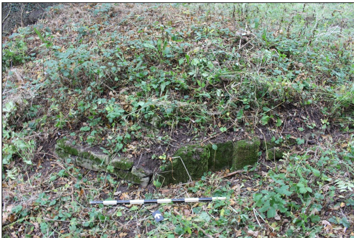
Plate 13: The visible remains of East sluice north wall. Looking northeast (L. Binns, 2016)
