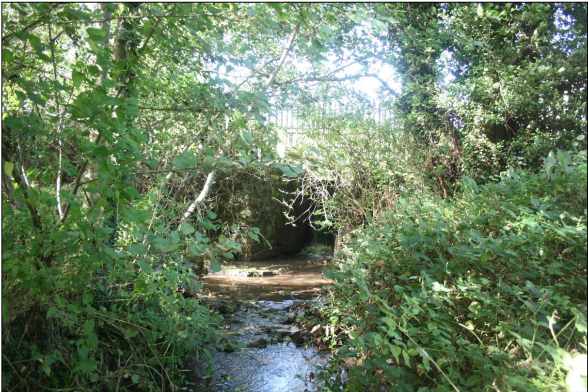
Plate 1: Sluice at the north end of the site in Upper Dam, looking north (L. Binns 2016)
