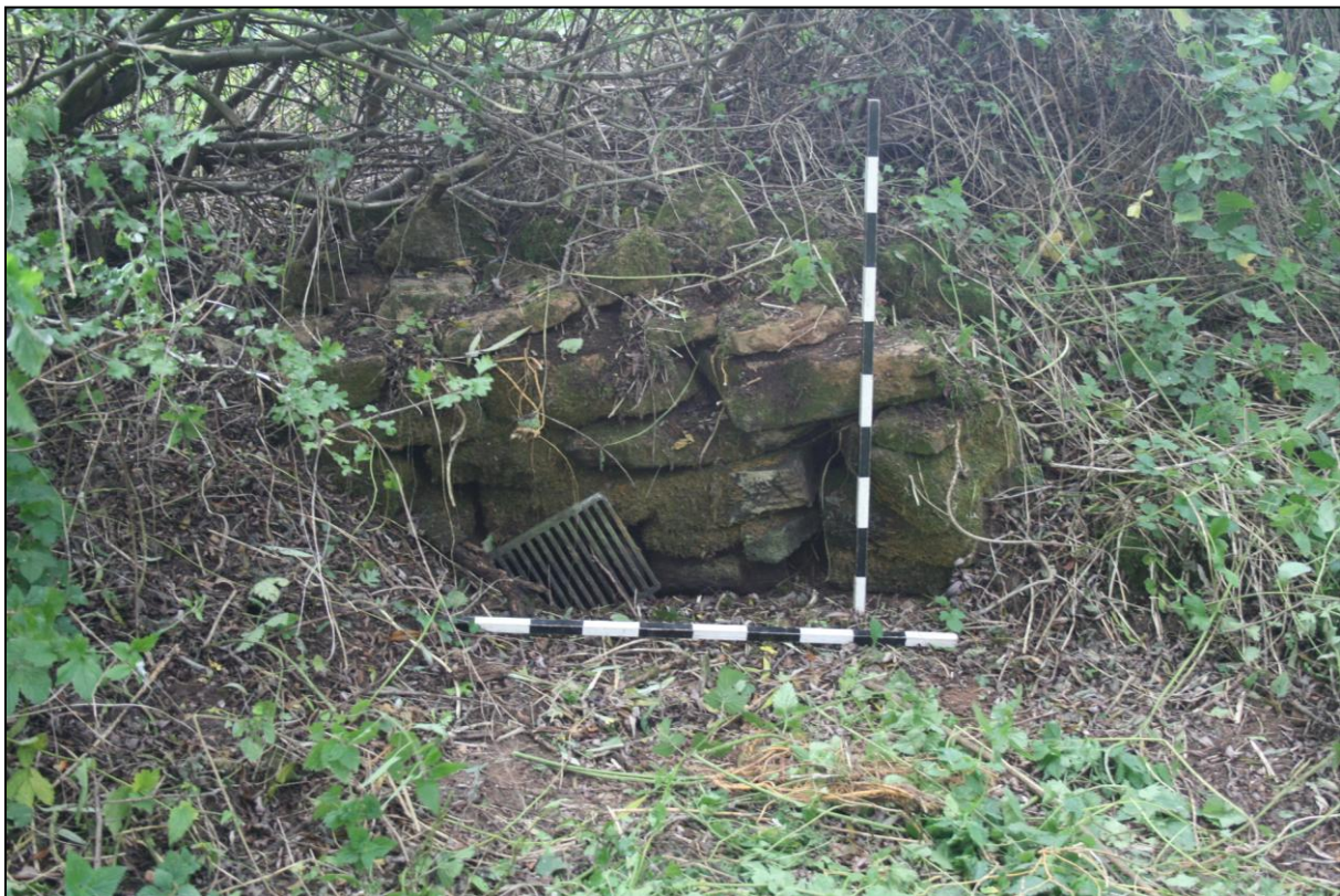
Plate 3: Drain found at the north west end of the site in Upper Dam, looking northwest (L. Binns 2016)
