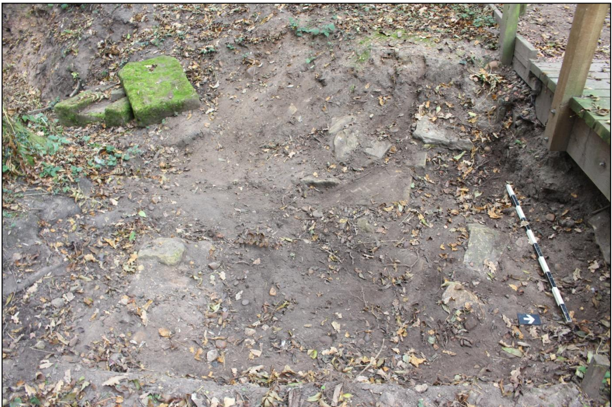
Plate 15: Loose stonework found north of Dam Banks south sluice Looking west (L. Binns, 2016)
