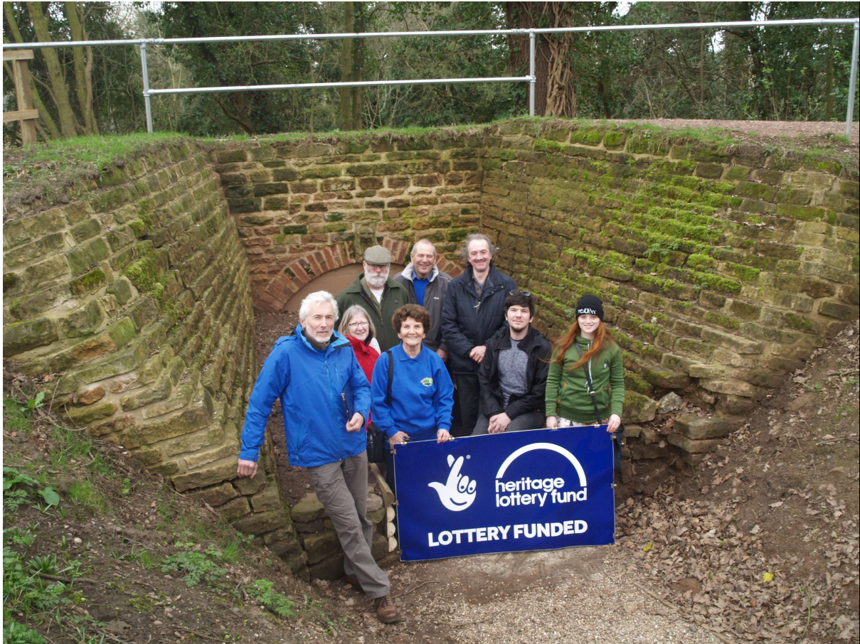
Grange Cottages Sluice, Papplewick – consolidation completed – March 2017
