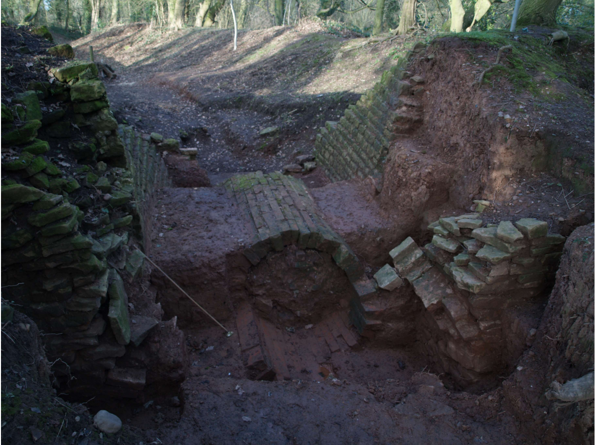
Grange Cottages Sluice, Papplewick - excavation completed - February 2015
