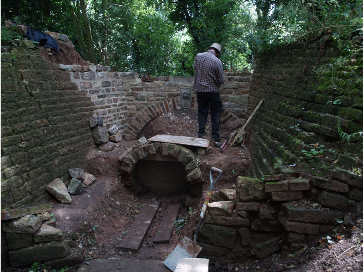
Grange Cottages Sluice, Papplewick – Consolidation underway - August 2015
