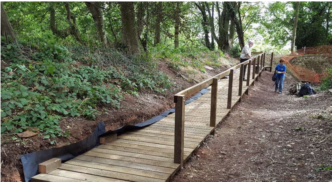
Grange Cottages Sluice, Papplewick – Construction of ramped access - Summer 2016
