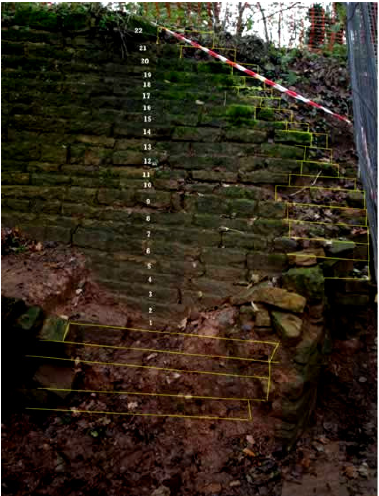
Figure 11: The west wall, facing west (November 2014), showing proposed conservation
