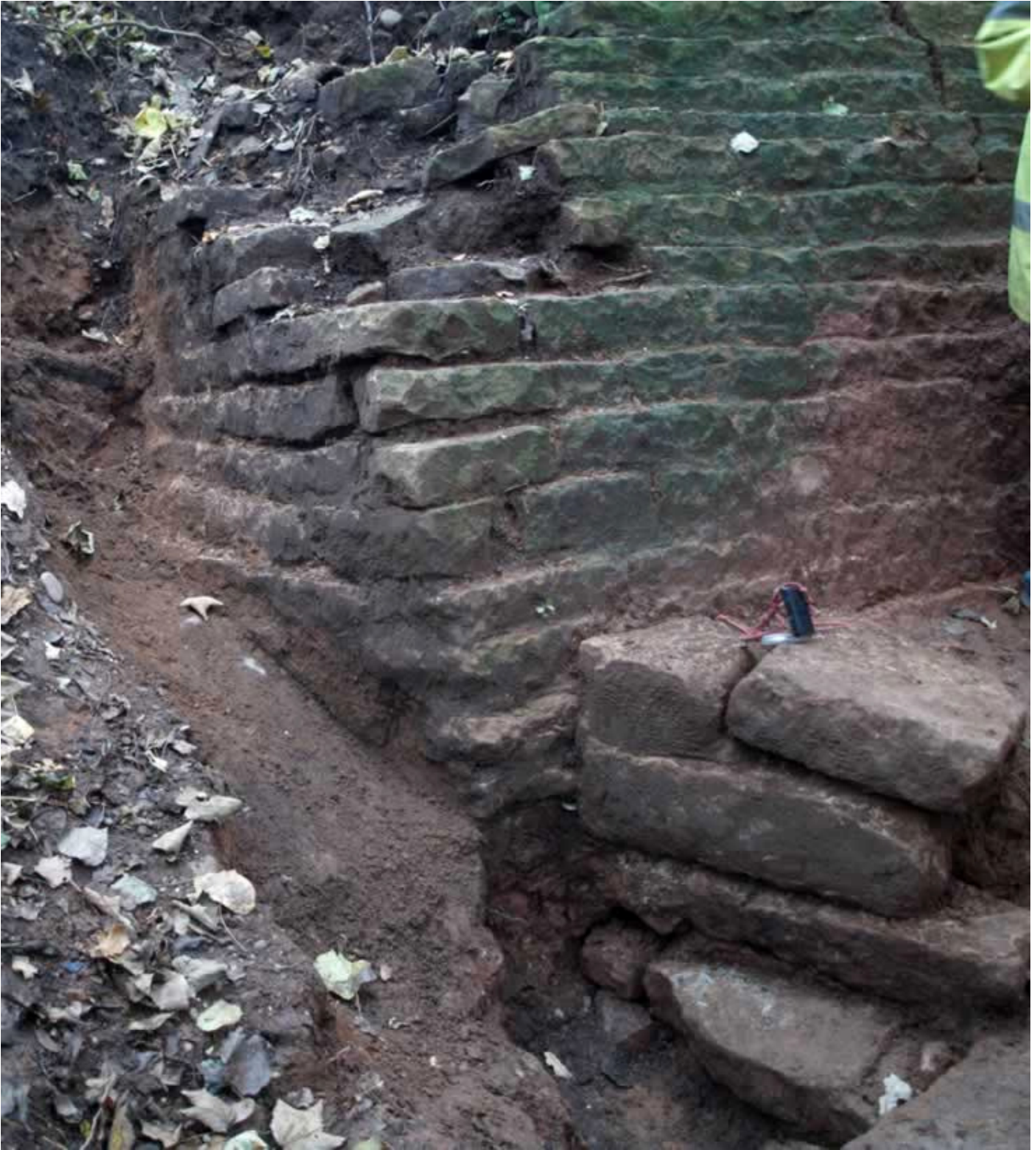
Figure 5: Detail of the northeast corner (November 2012)
