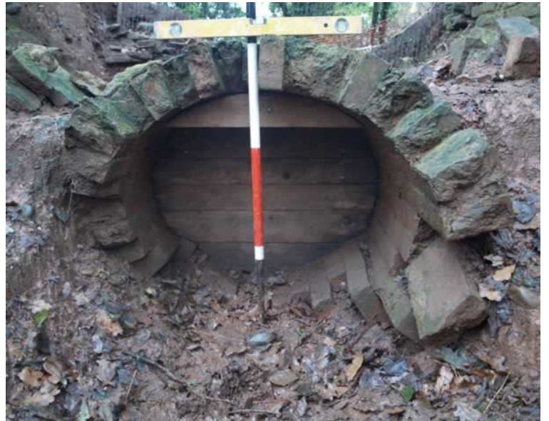
Figure 2: Detail of the brick tube (November 2014)
