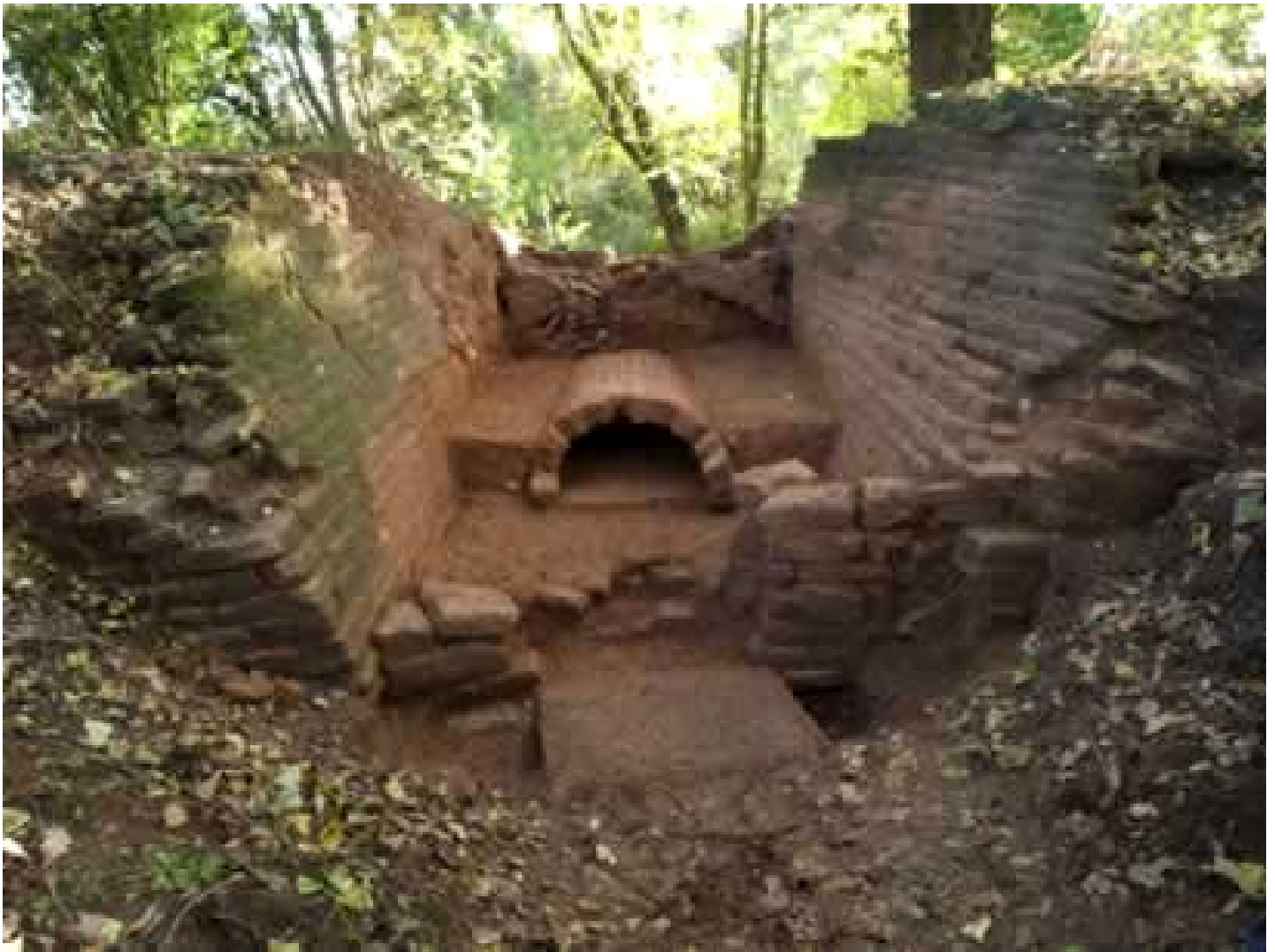
Figure 1: The sluice, looking south (November 2012)
