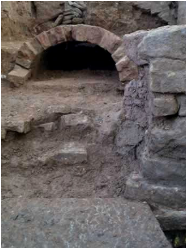
Figure 3: Detail of the wall at the northwest corner (November 2012)
