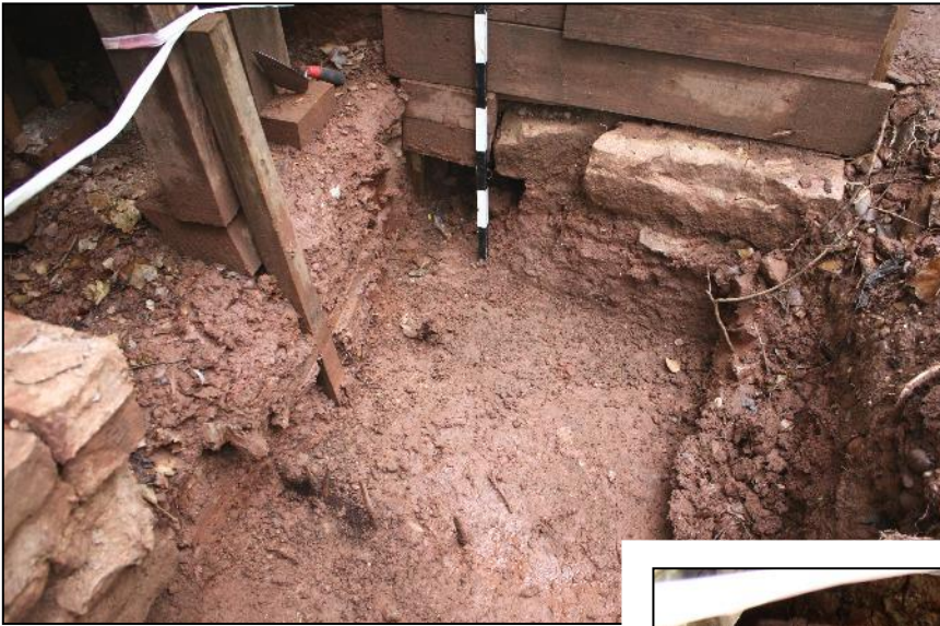
Plate 8: Iron nails of former wooden drain, shute or launder, here exposed at low level outside wall entry.
