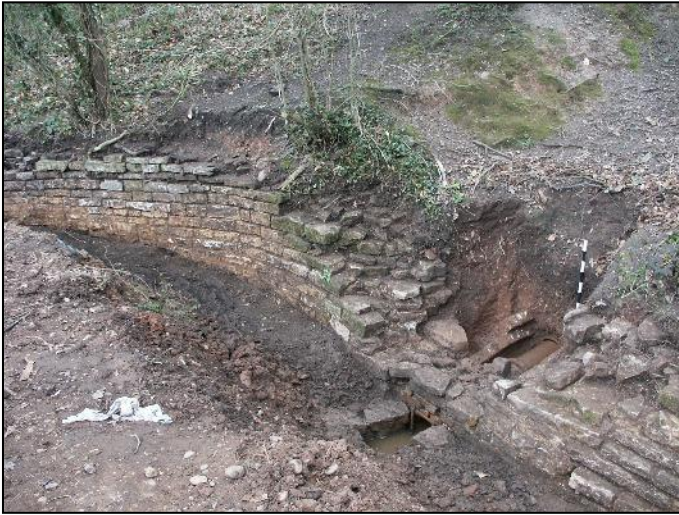
Plate 26: Length of walling showing on the south-west inner edge of Moor Pond.
