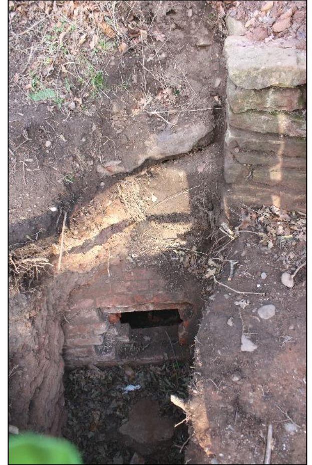
Plate 17: Entry subsequently made into side of brick drain (see Plates 20-22).
