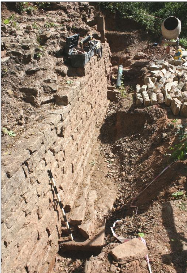
Plate 13: View looking eastwards along the west part of the walled feature, showing projecting foundation stones.
