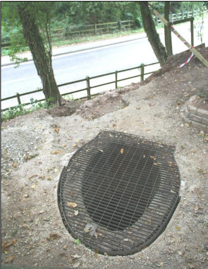
Plate 24: Rebuilt top (with safety grill) of the water control feature, situated behind the wall on Papplewick Lane.
