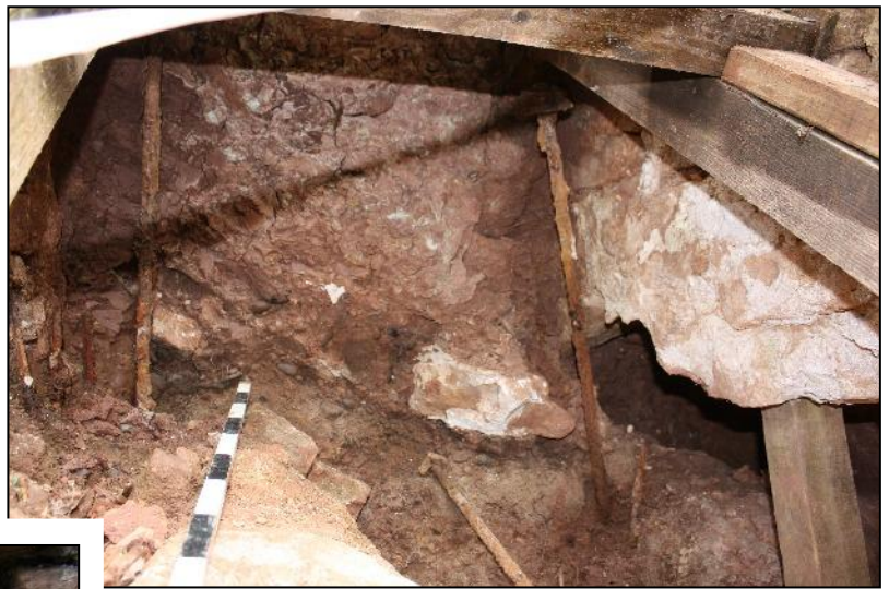
Plate 9: Two lines of metal rods and nails showing high up and well within the wall entry.
