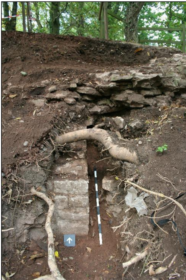
Plate 2: The west corner of a former opening showing beneath a tree root.
