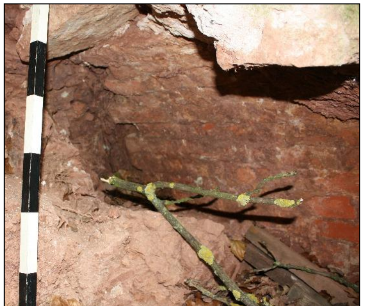
Plate 11: More intact east side of the brick drain, here overlain by extended stonework.
