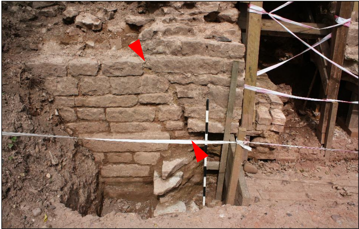
Plate 12: Intact stonework on left (west) side of the central entry, with part of brick arch showing to the right. The arrows indicate a break or change in the stonework.
