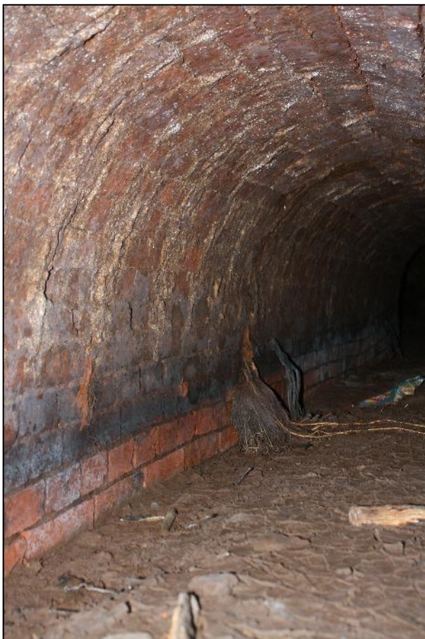
Plate 20: View of internal side walling of arched brick drain, looking east from a point near the south-west corner of the wall near Papplewick Lane.
