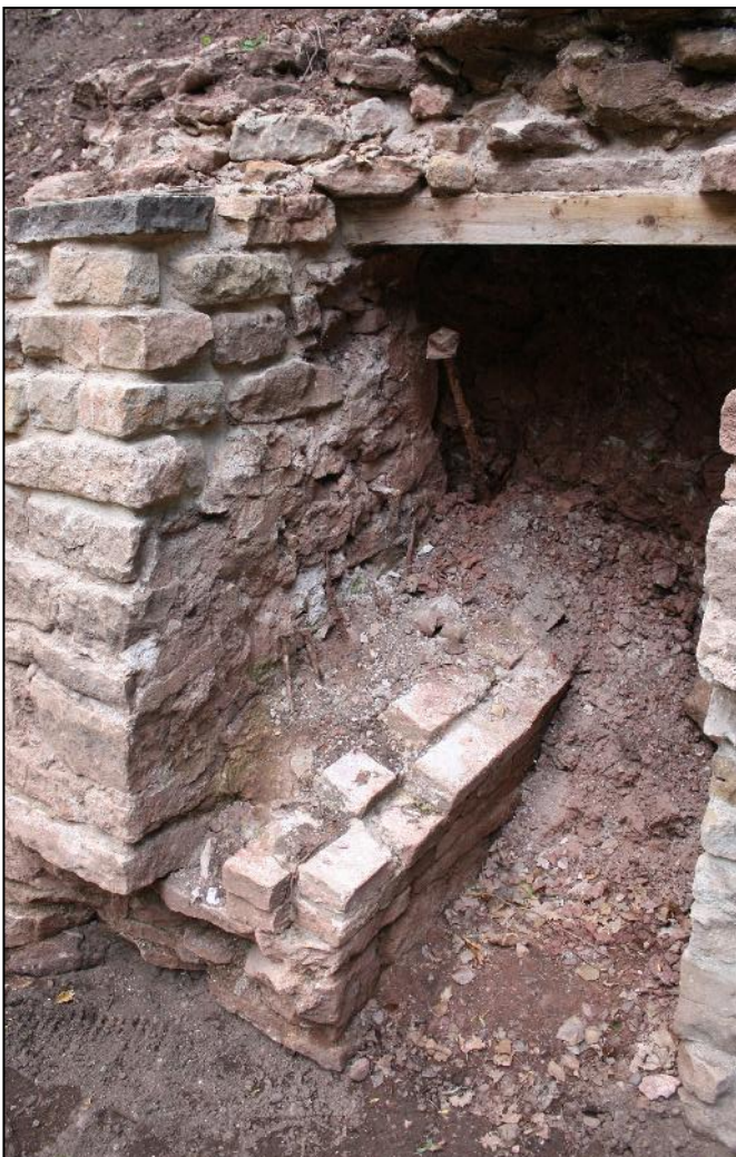
Plate 10: Surviving west side of former brick drain extending back into the wall entry.
