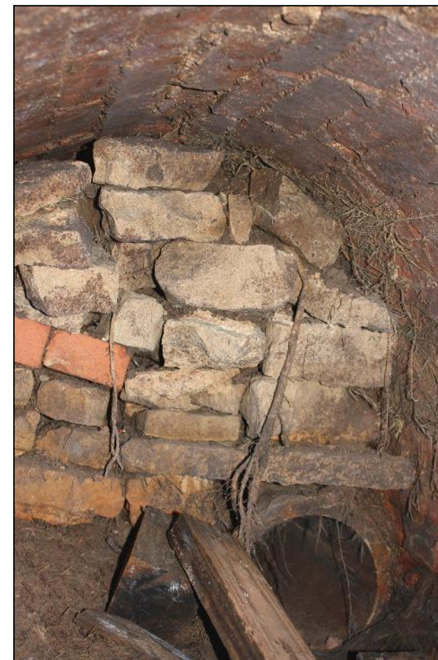
Plate 22: View looking west showing stone and brickwork blocking and ceramic drain.
