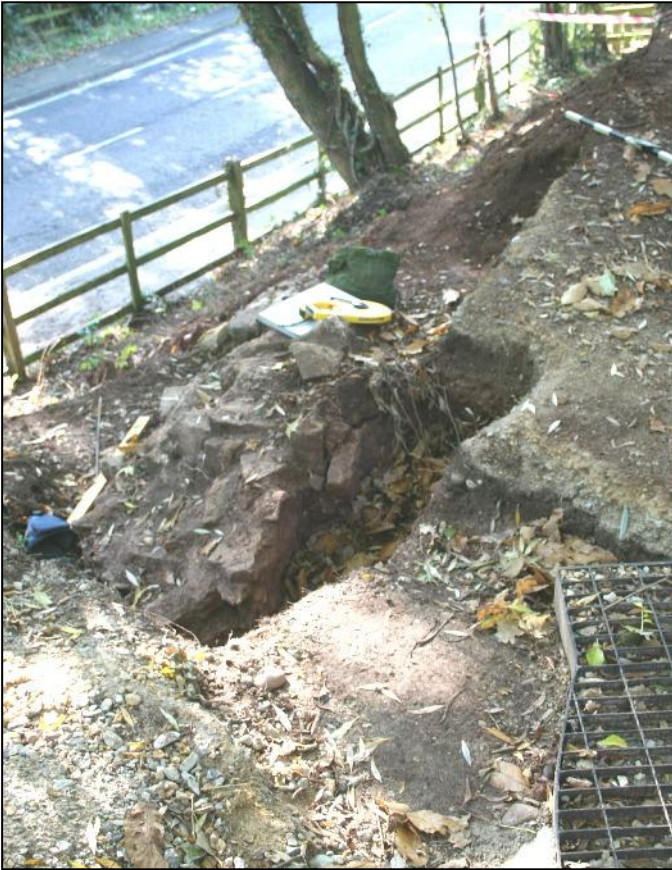
Plate 23: View of the north, rear side of the wall's core stonework.
