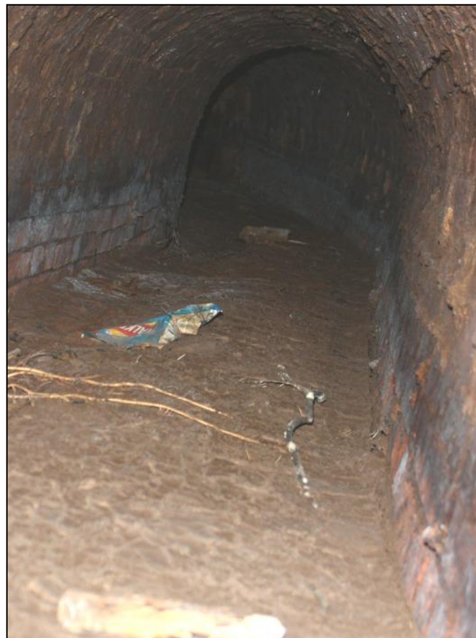
Plate 21: Another view showing change of direction of drain as it continues towards the water control feature.
