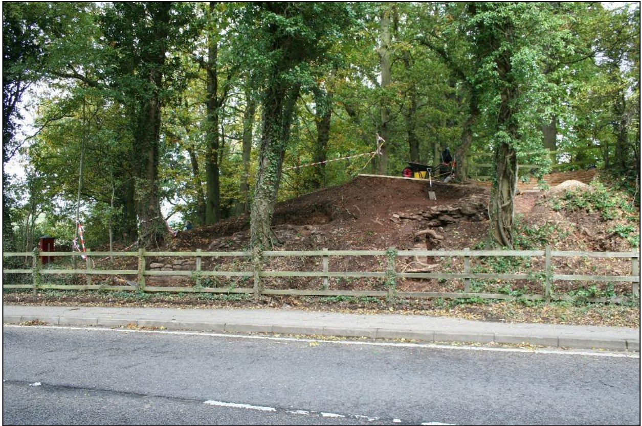
Plate 1: Excavations of a previously hidden wall underway on the north side of Papplewick Lane, October 2009.
