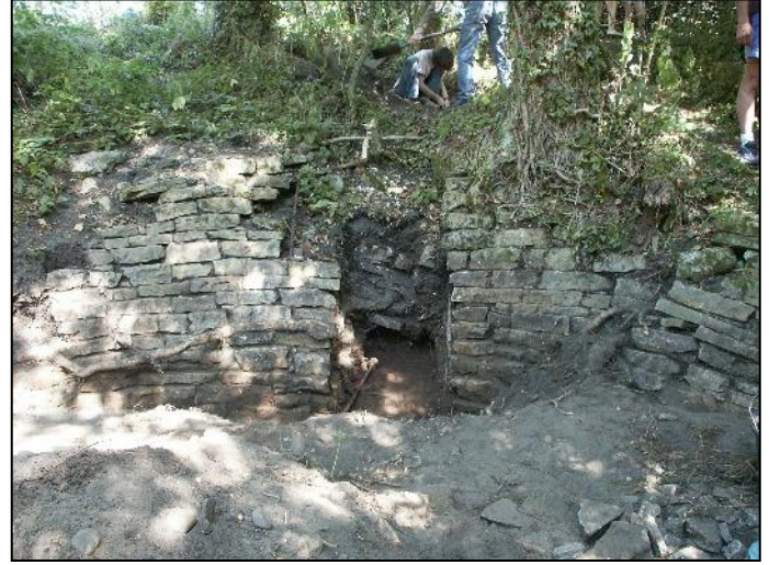
Plate 27: Length of walling with narrow central opening showing on the east inner side of Moor Pond.
