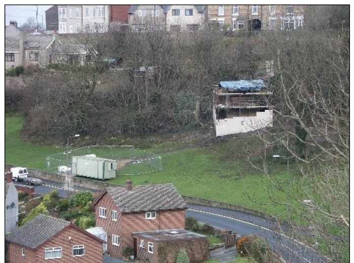
Plate 30: View taken from the Fountain Garden wall showing Hockley and the Cundy House surrounded by scaffolding during its restoration in 2002-03.
