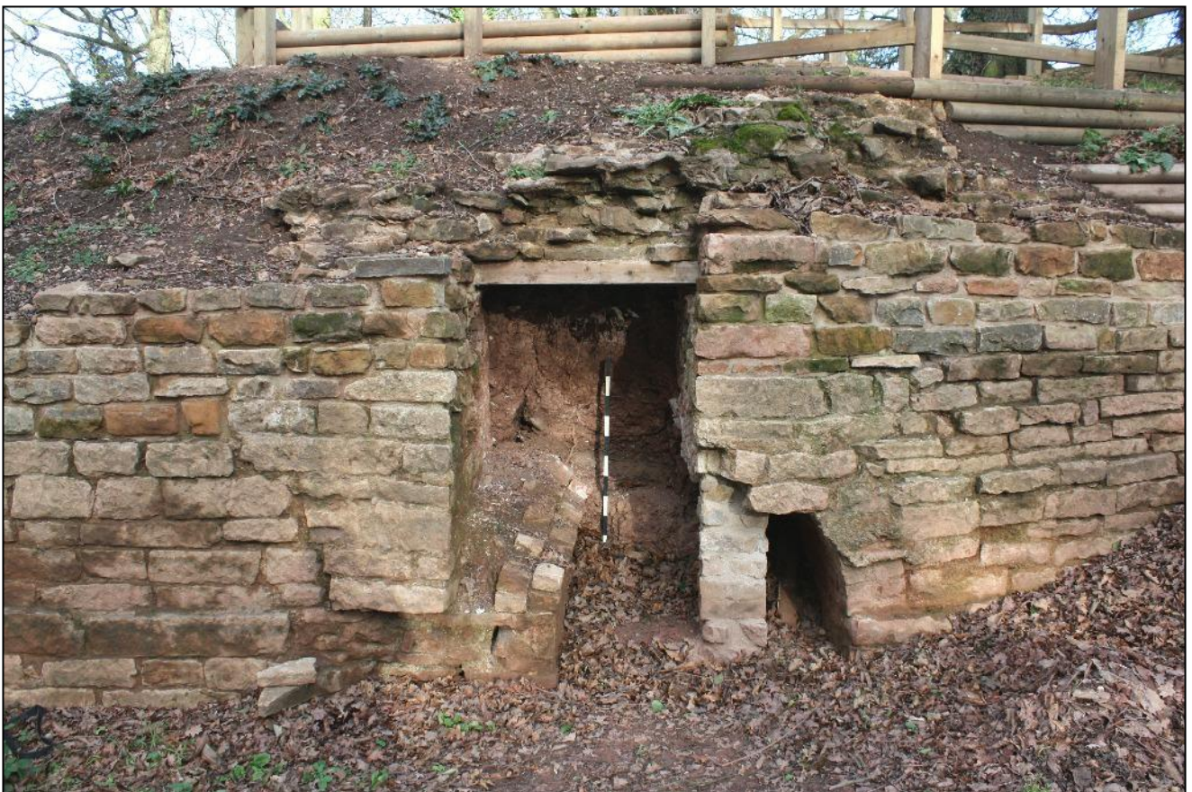
Plate 19: The central entry with more of the brick arch showing, along with an added support timber and a brick pillar.
